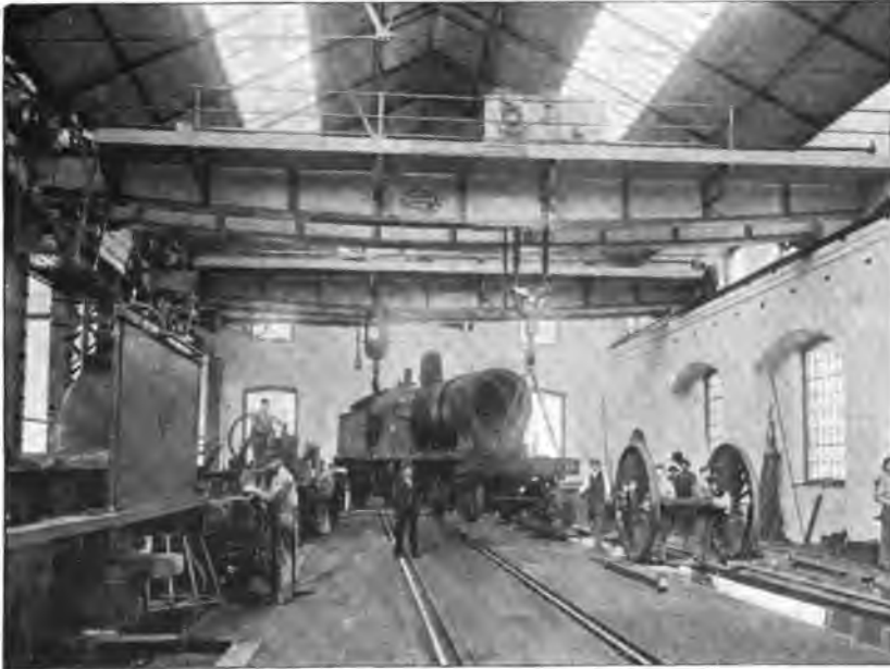
ERECTING SHOP, ISLINGTON.
